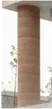
rammed earth columns (earth colour)
