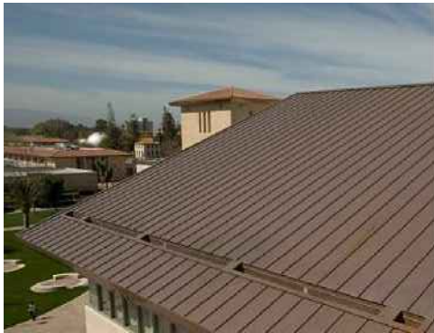
metal roof sheeting (copper)
